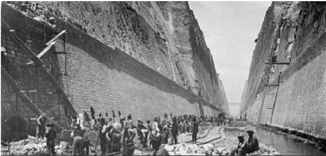
Isthmus Photo during Construction
