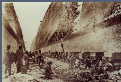
Photo of Construction Works
