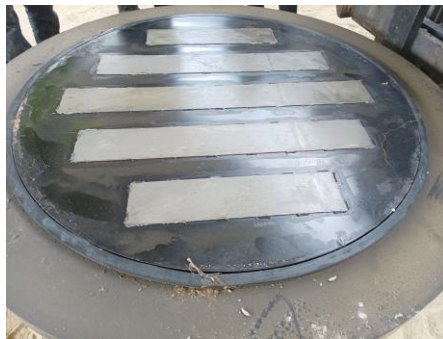
Sliding Material of Pot Bearings
