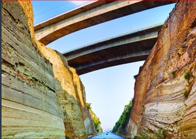
Bridge View from Water Level
