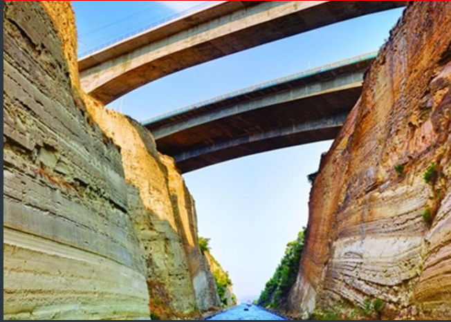
Bridge View from Water Level
