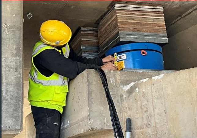
Hydraulic Jacks with Load Distribution Plates
