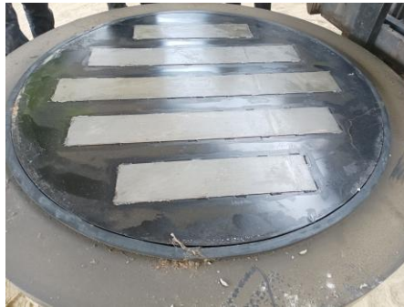
Sliding Material of Pot Bearings
