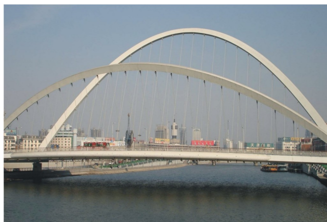
DAIKOU BRIDGE, MAIN SPAN:250m, Hanging Cable:BHC73W5.
