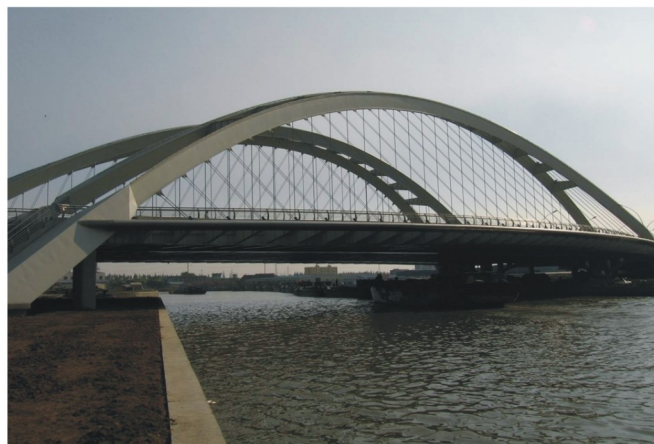
ETSUKAWA BRIDGE, Main Span:329.54m, Hanging Cable:AHC73W5.
