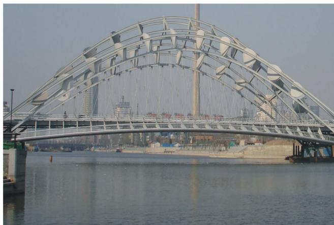
Bouka Bridge, Main Span:250m, Hanging Cable:CHC37W5, CHC73W5
