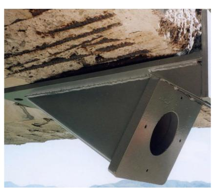
Placement of steel tube and anchoring plate
