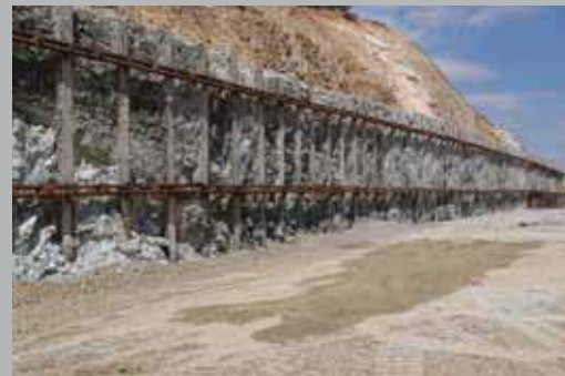
Retaining wall with temporary anchors
