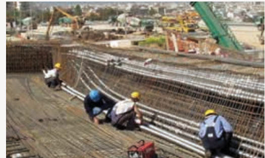
Fig.2 Recommended Ducts Arrangement
